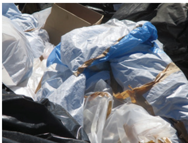
Figure 17: Poorly controlled asbestos waste at licenced tip (author's own photo approx 2015)
