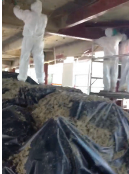
Figure 12: Confidential image provided by a respondent of licenced removal work involving limpet asbestos
