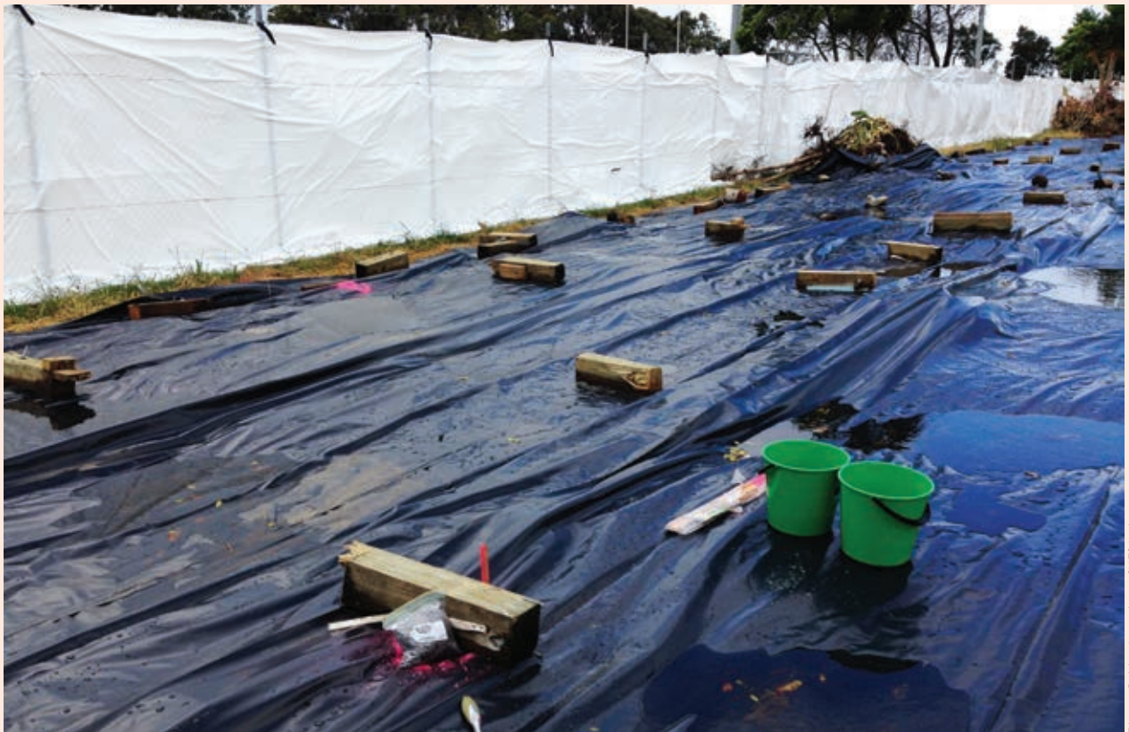
Figure 27. Temporary cover of contaminated soil.
